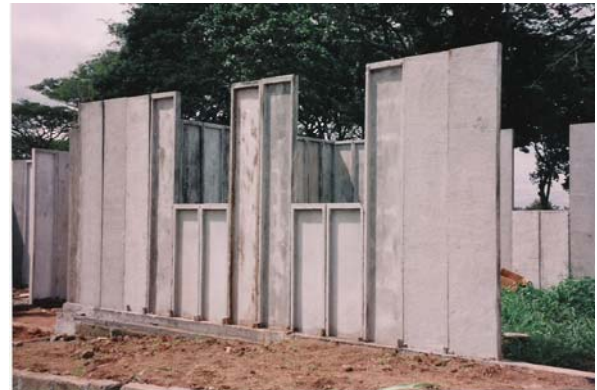
Placing the walling elements on U-beams
