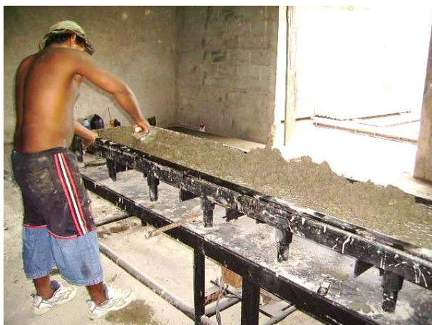
vibrating the panels
